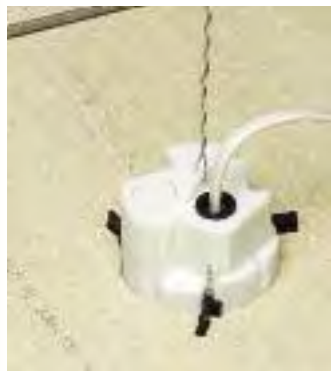
4 Choose the appropriate knockout (1/2" or 3/4"). Install supplied NM cable connector. Pull cable.
