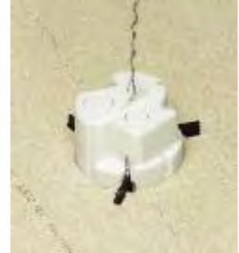
3 Attach drop wire to loop. Attach to framing member for 50 lb rating.
