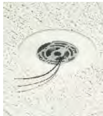
5 FL430, ready for installation of fixture or detector.
