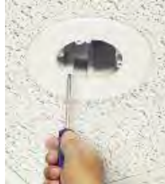
2 Align fixture as necessary. Tighten mounting wing screws.
